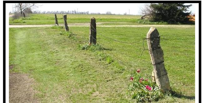
The holes for the posts were dug by hand every 15 feet to a depth of 24+ inches. There were about 320 posts per mile.
