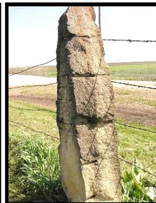
*The limestone known as post rock has had many uses other than for the construction of fence posts. The material's durability makes it an excellent building material.*
